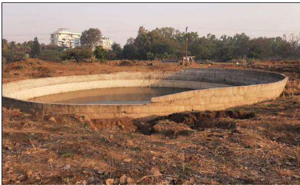
Plate No. 3.2 Construction of new well near Gymkhana
