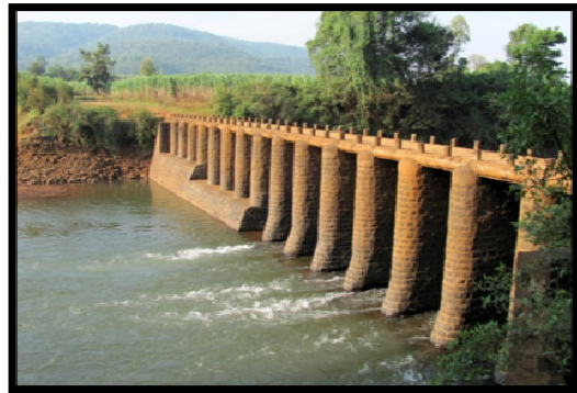
c) Dam Under construction on Dhamni river d) A typical Kolhapur Type (K.T.) weir
