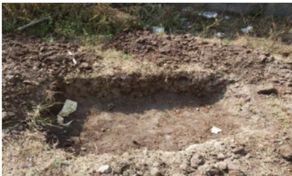
Figure-3. Step 1 of pilot scale model of horizontal flow constructed wetland.
