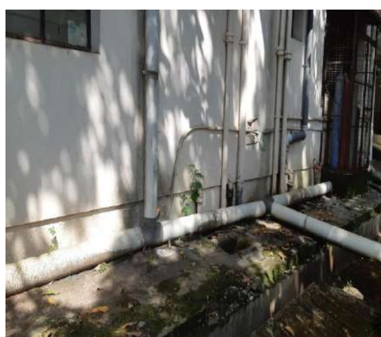
Plate: 3.6. Roof top rain water harvesting at Department of Environmental Science.
